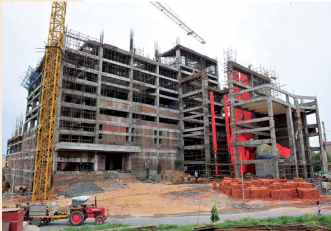
Work in progress: 120 MTPD dairy whitener plant at Banaskantha.
