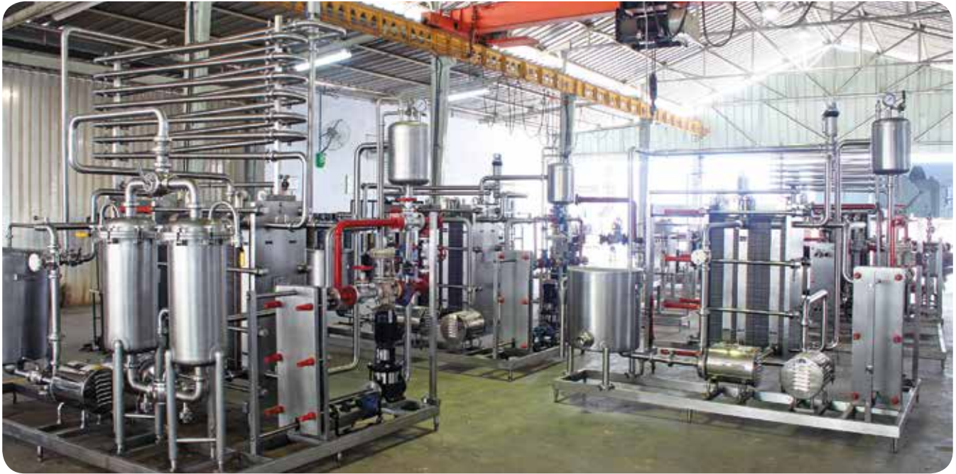
PHE assembly facility
